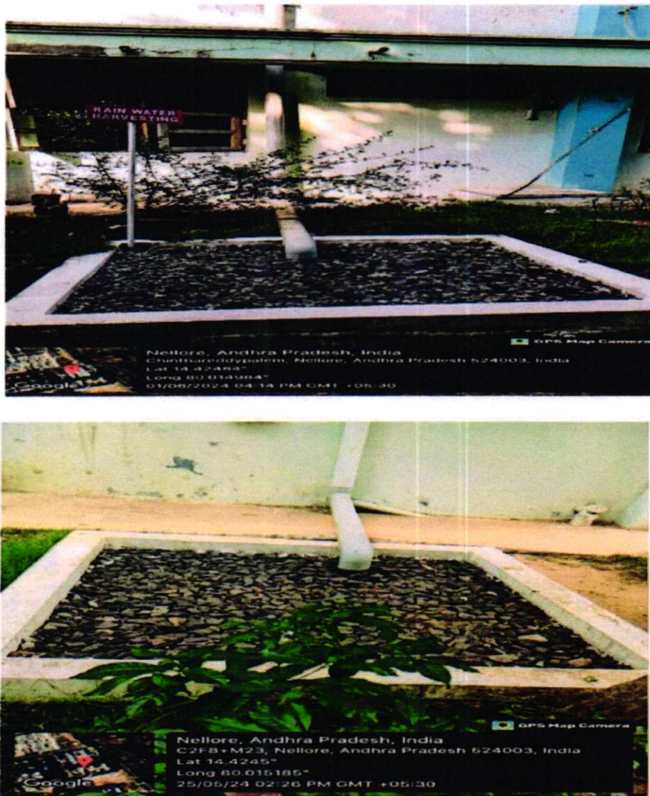
Fig.1: Rain Water Harvesting (RWH) system implemented in the College
